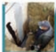
Crack Repair
