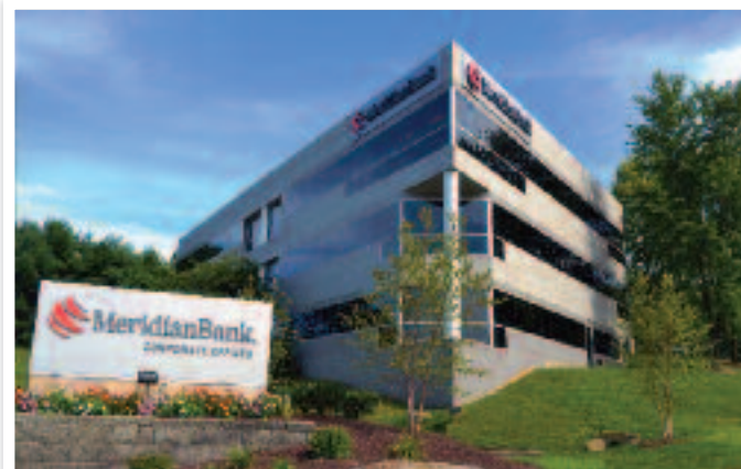
To accommodate its growth, Meridian moved to a new Corporate Headquarters in Malvern PA in 2013.
