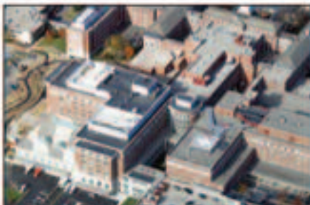
Reading Hospital Building N
