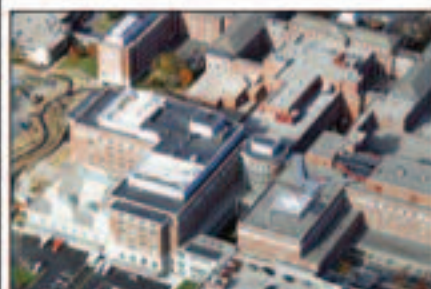
Reading Hospital Building N
