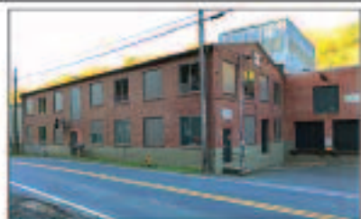
BOYERTOWN INDUSTRIAL BUILDING
