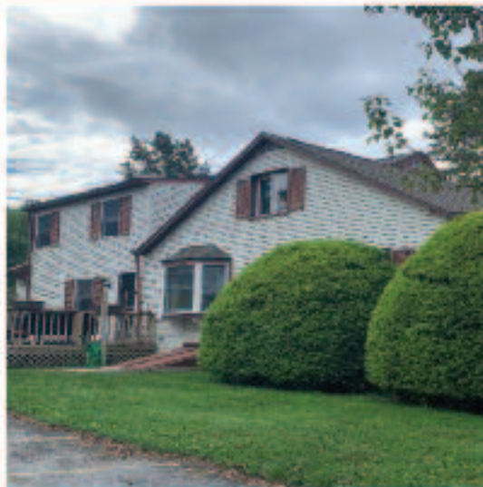
MIXED USE PROFESSIONAL BUILDING ON E. HIGH ST. IN THE BOROUGH OF POTTSTOWN.
