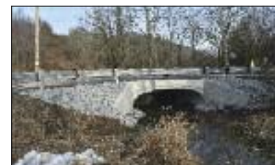
Emergency bridge replacement.
