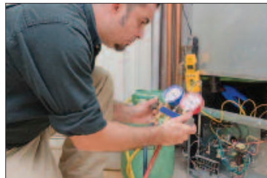
HVAC - Residential, Commercial & Industrial
